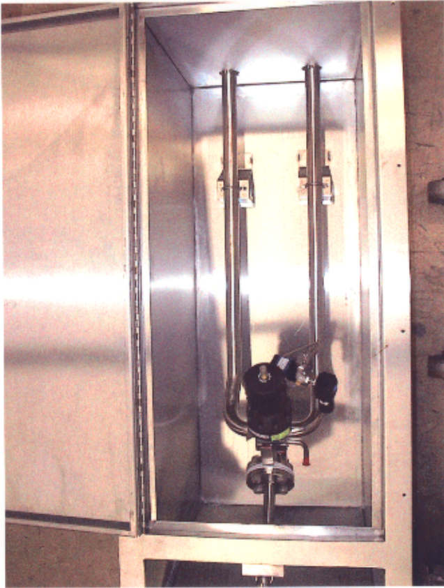
WFO Station - Sanitary Approved Welds
